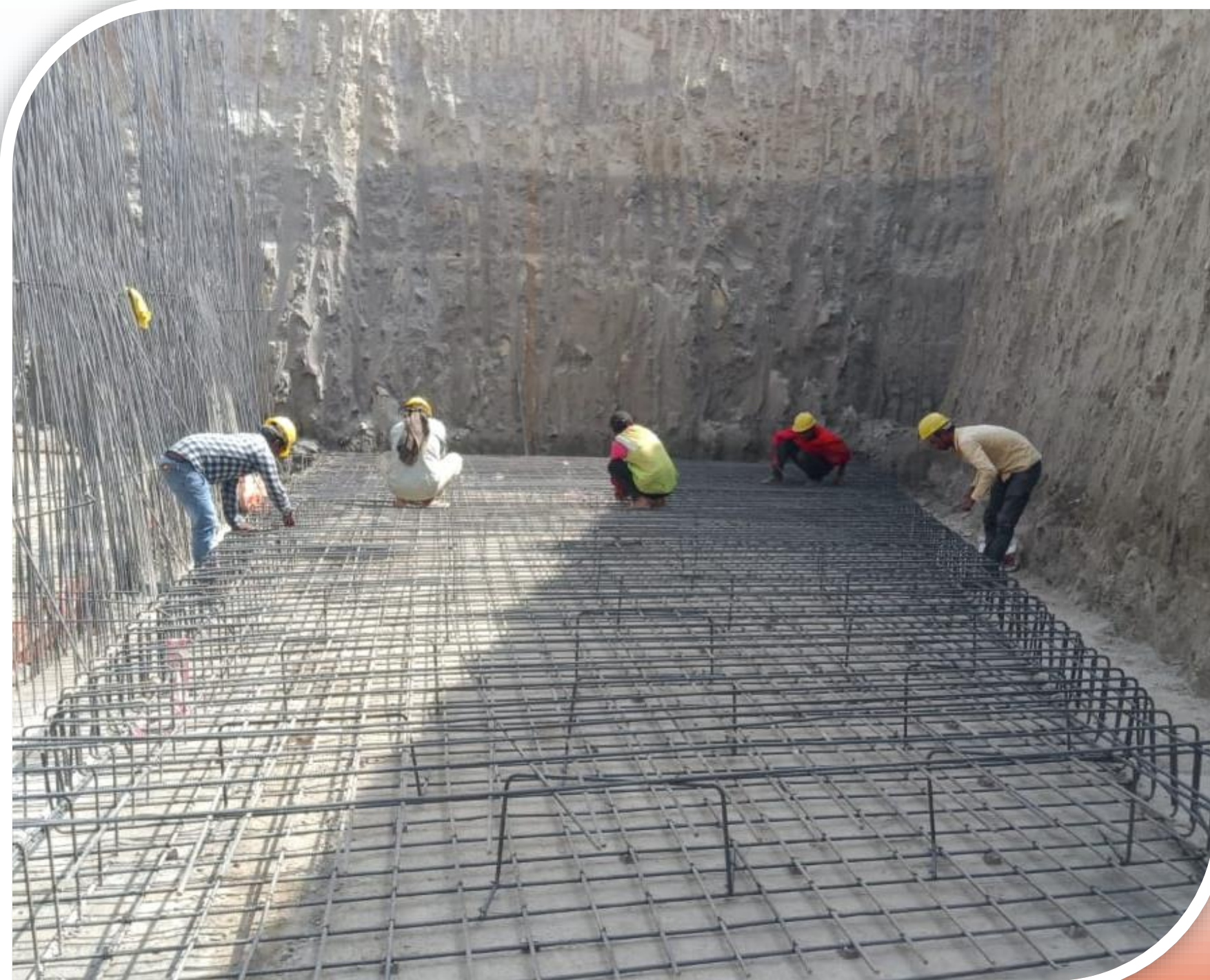
STP raft steel binding in progress
