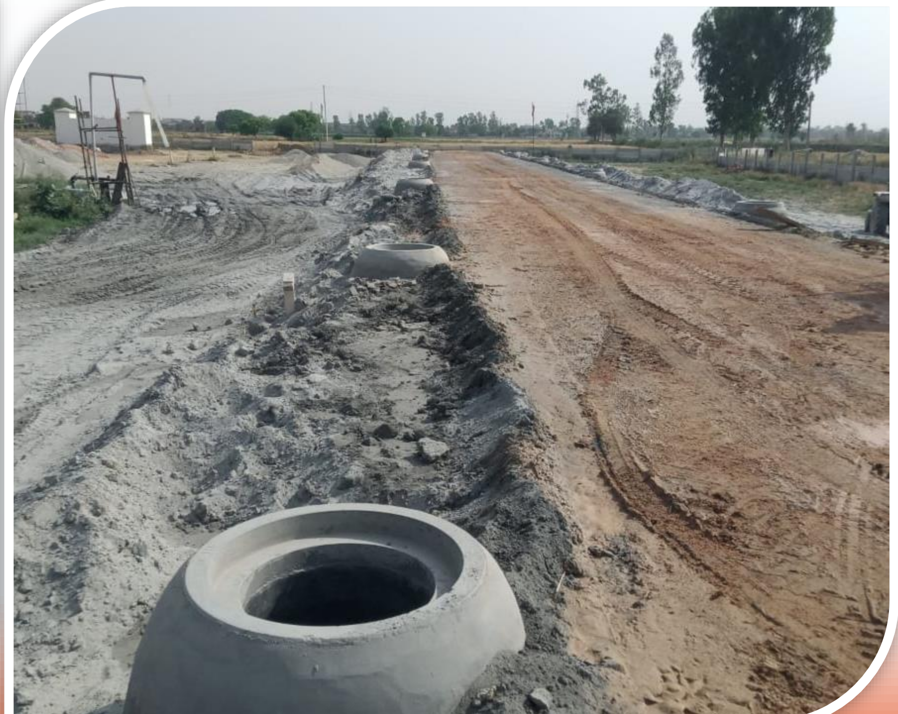
Sewage line & Manhole work completed
