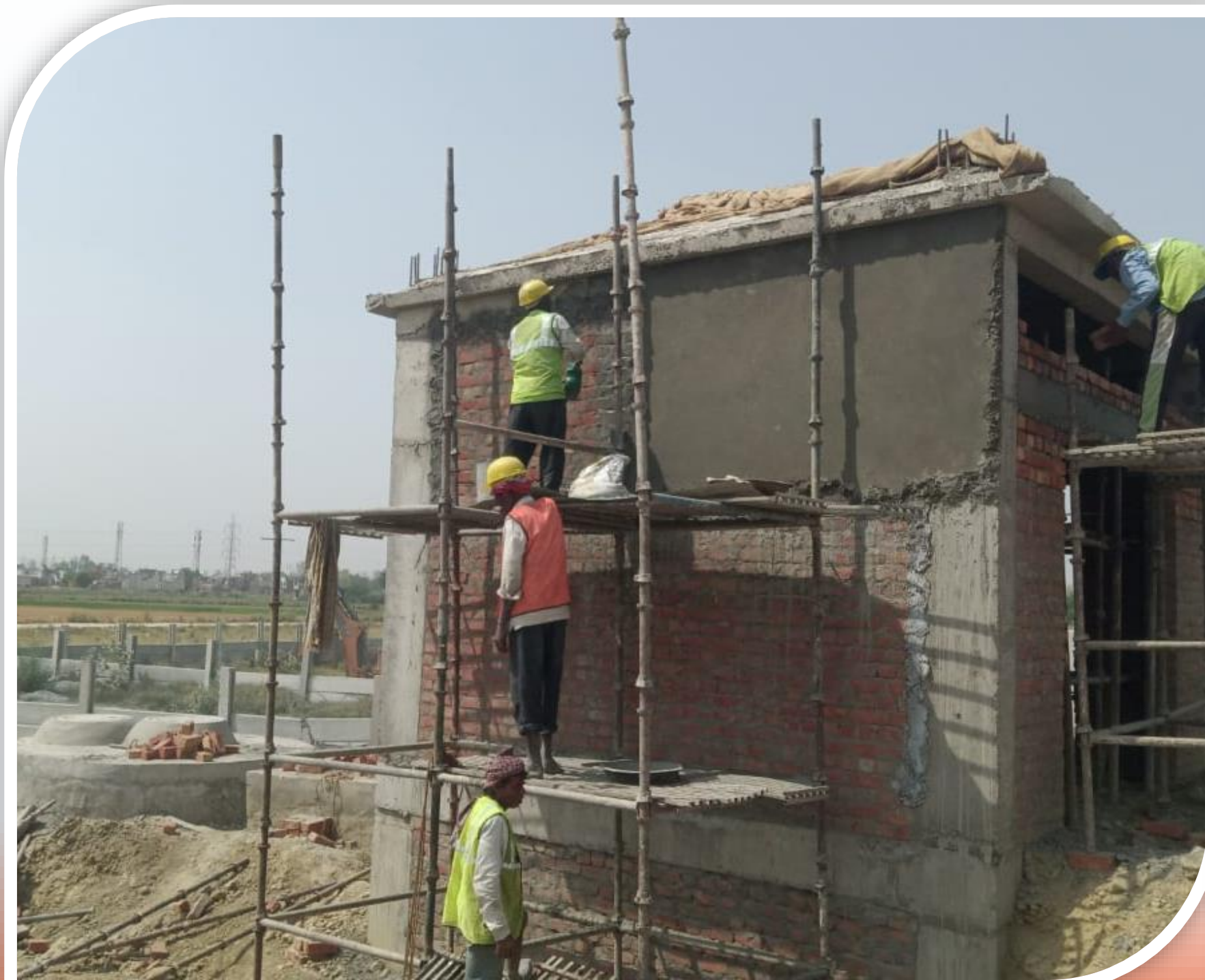
Milk/Vegetable Booth plaster work in progress
