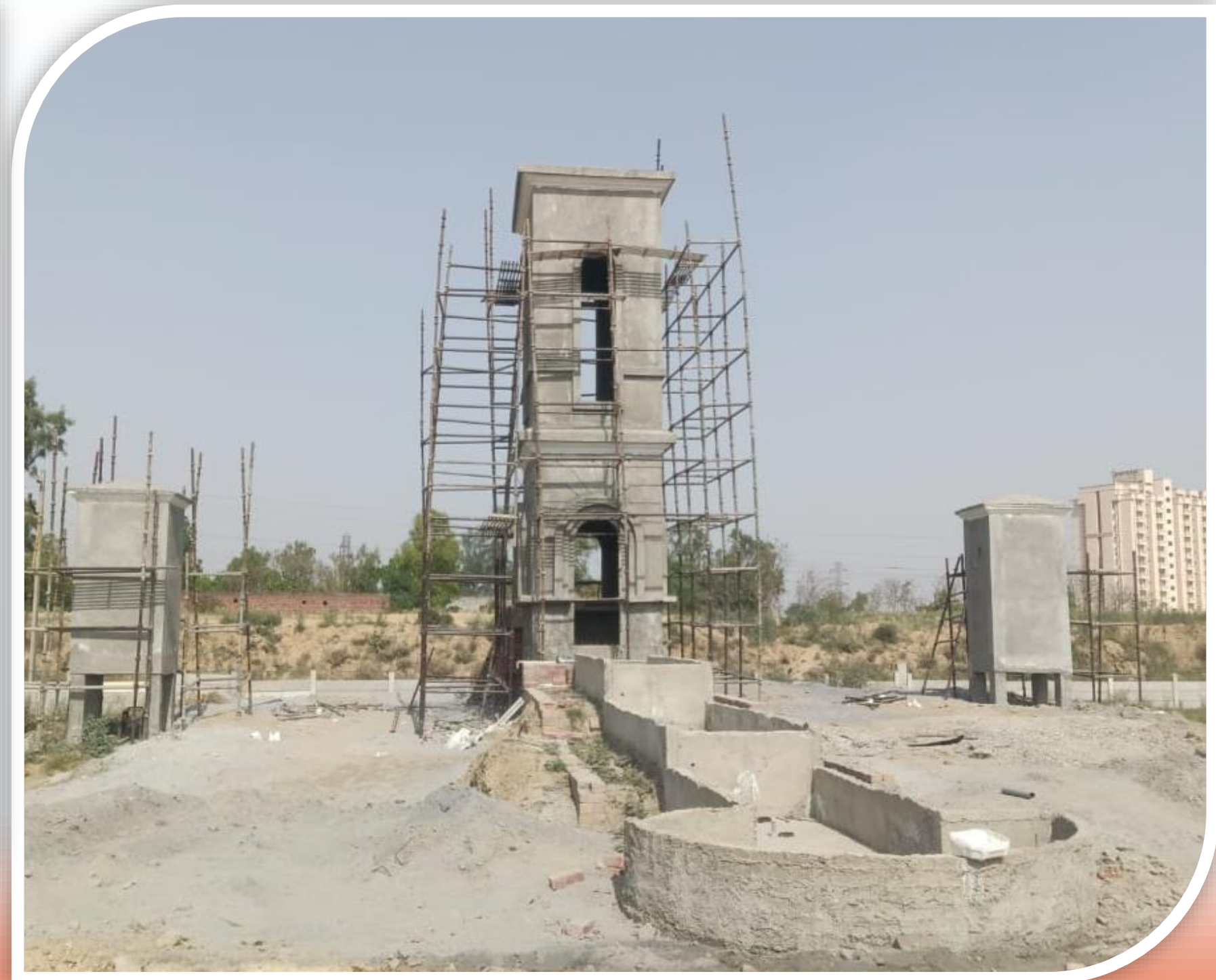
Entrance Gate-2 external plaster completed
