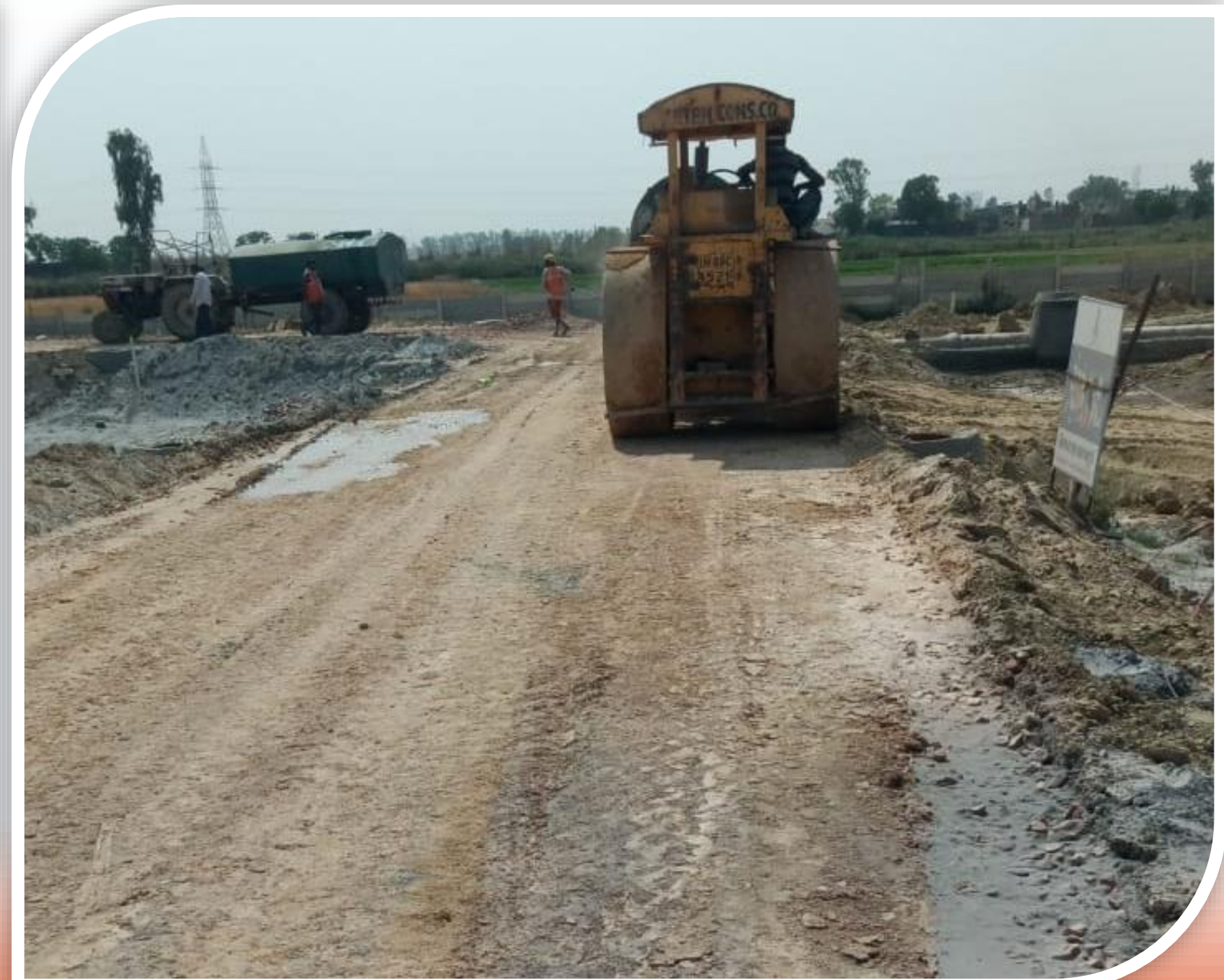
Road water bond macadam work in progress
