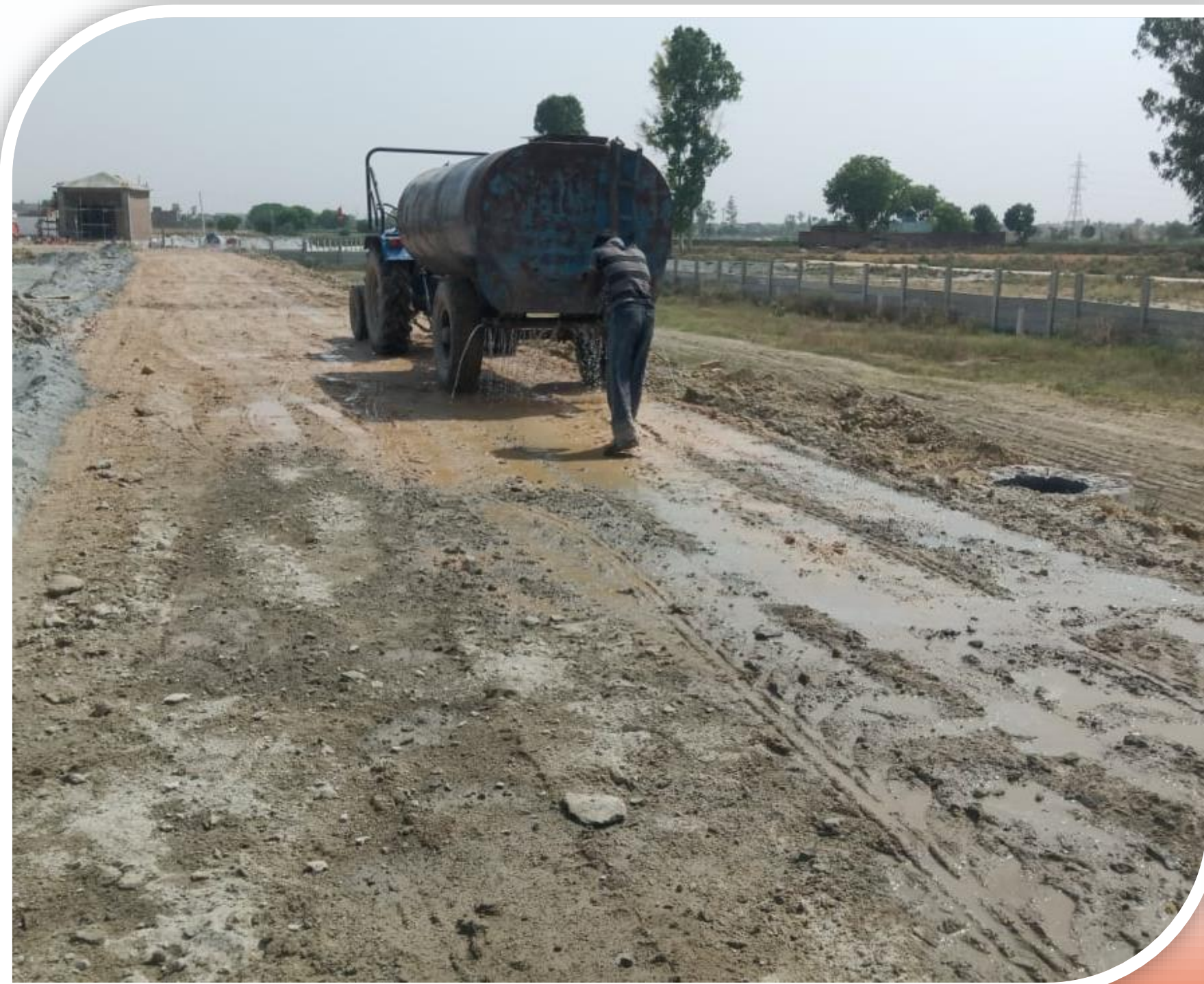
Road water bond macadam work in progress
