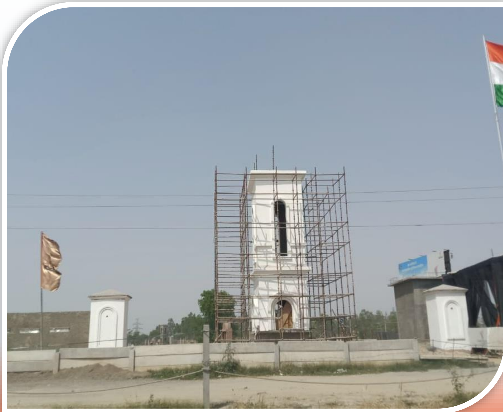
Entrance Gate-1 external paint in progress
