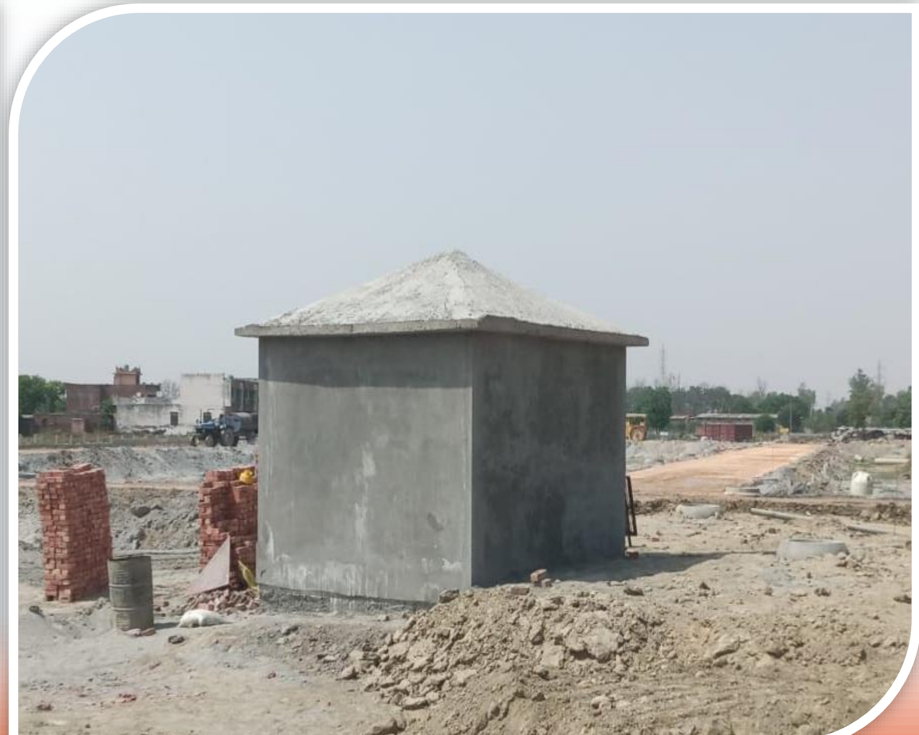
Pump room plaster work completed
